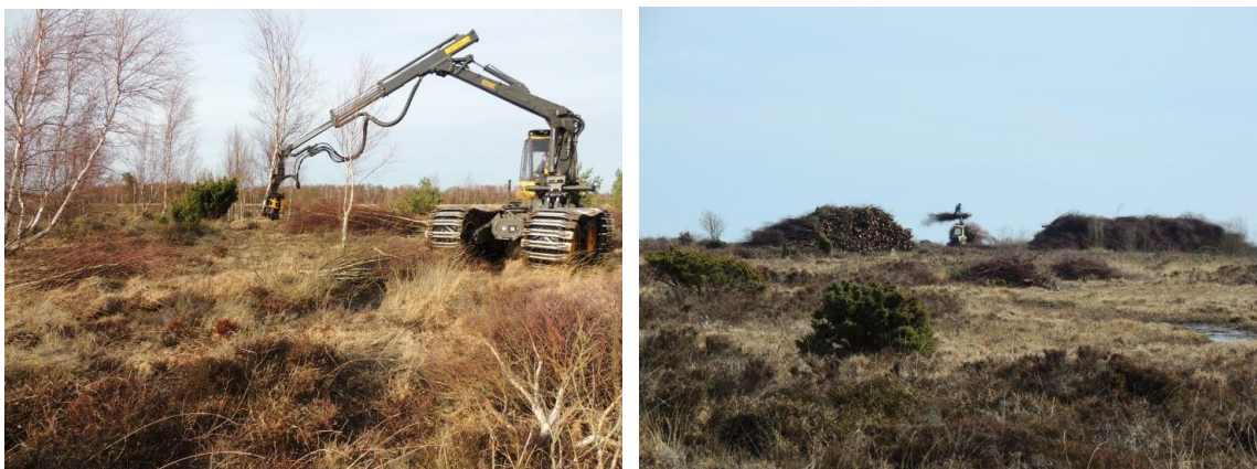
Clearing of trees with special machines for wet conditions
